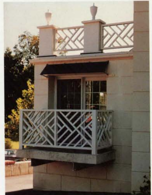
Custom Railing For Office Building Westport, CT.
