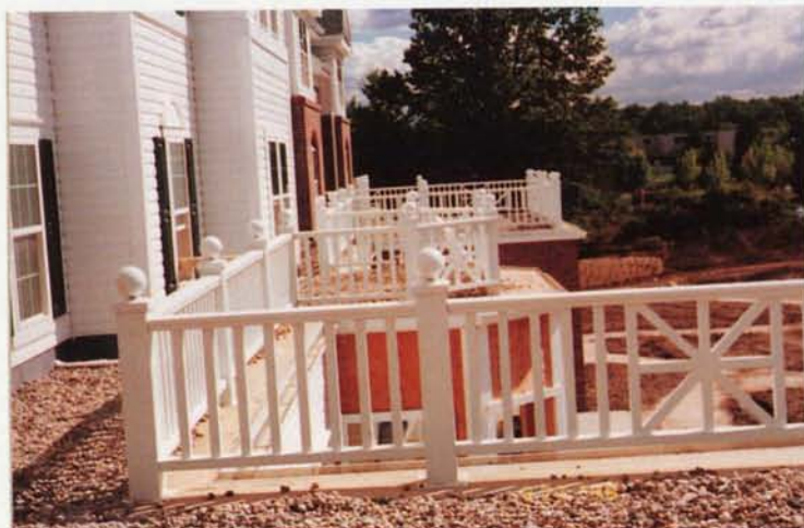
Custom Railing For Brighton Gardens Westlake, OH.
