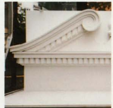
Historic Cornice Reproduction
