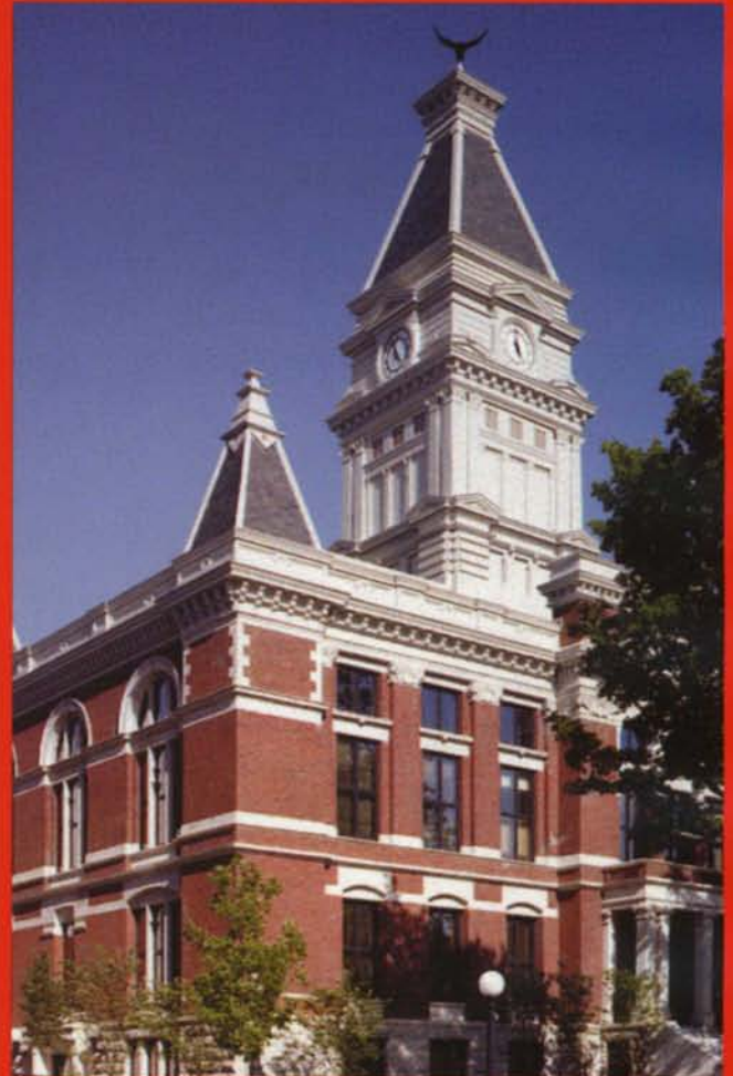
Montgomery County Courthouse Clarksville, TN Lyle-Cook-Martin, Architects Clarksville, TN
