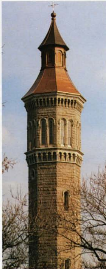
High Bridge Tower New York, NY William Hall Partnership New York, NY
